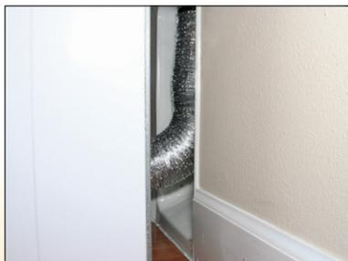
Extends and compresses smoothly while maintaining 4" inner diameter.
